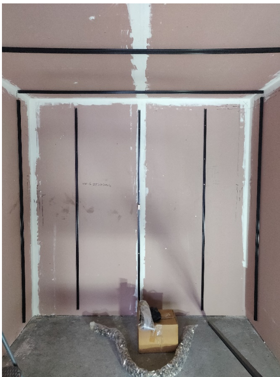
SPECIMEN RAILS INSTALLATION
