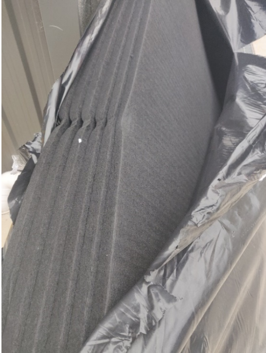
FIGURE 3: INSULATION APPLIED AT THE CEILING
